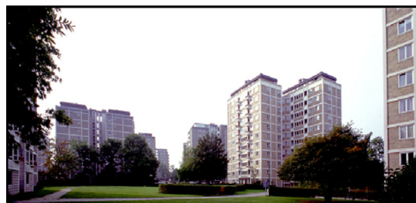
Bellahøjhusene, by Kristensen, Heiberg, Buhl, Larsen, Fink and Petersen, Denmark, 1951-1956.
